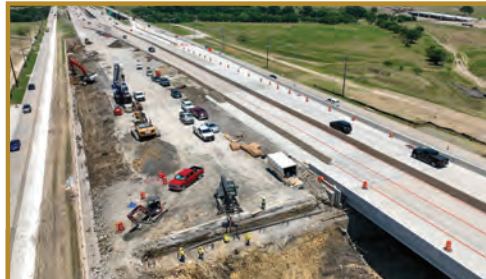
HNTB's drone photography of the DNT Widening construction in Frisco.
