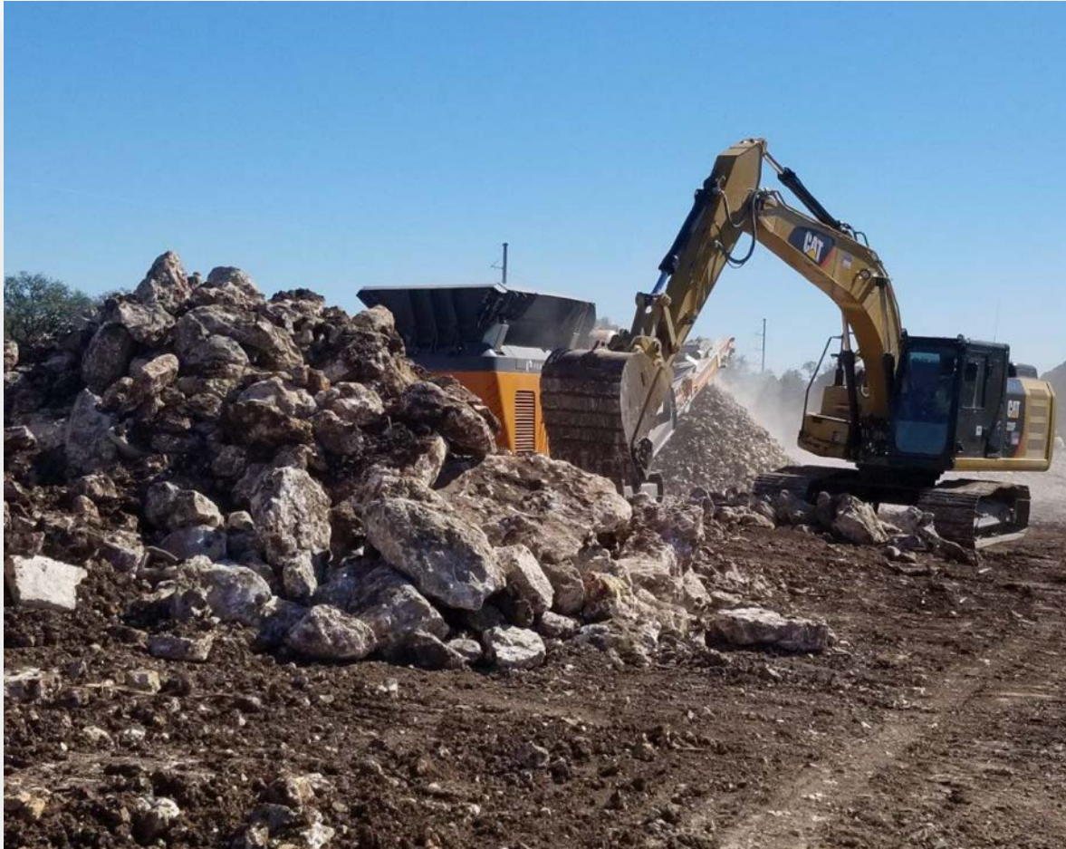
Rock crushing and material sorting operations on 45SW
