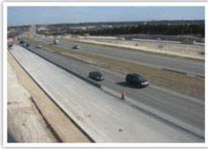
Paving has begun on the westbound frontage road.
