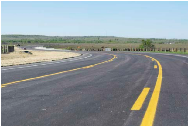
Final Kellam Road open to traffic
