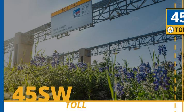
45SW Toll is a new 3.6-mile toll road with two lanes in each direction connecting MoPac eastward to FM 1626 in Hays County. The greenfield project is a new alignment that includes an at-grade intersection at FM 1626, an overpass at Bliss Spillar Road, and an interchange at MoPac. The project was built within existing TxDOT right-of-way with support from TxDOT, as well as Travis and Hays counties. Construction began in November 2016 and was completed in 2019.
