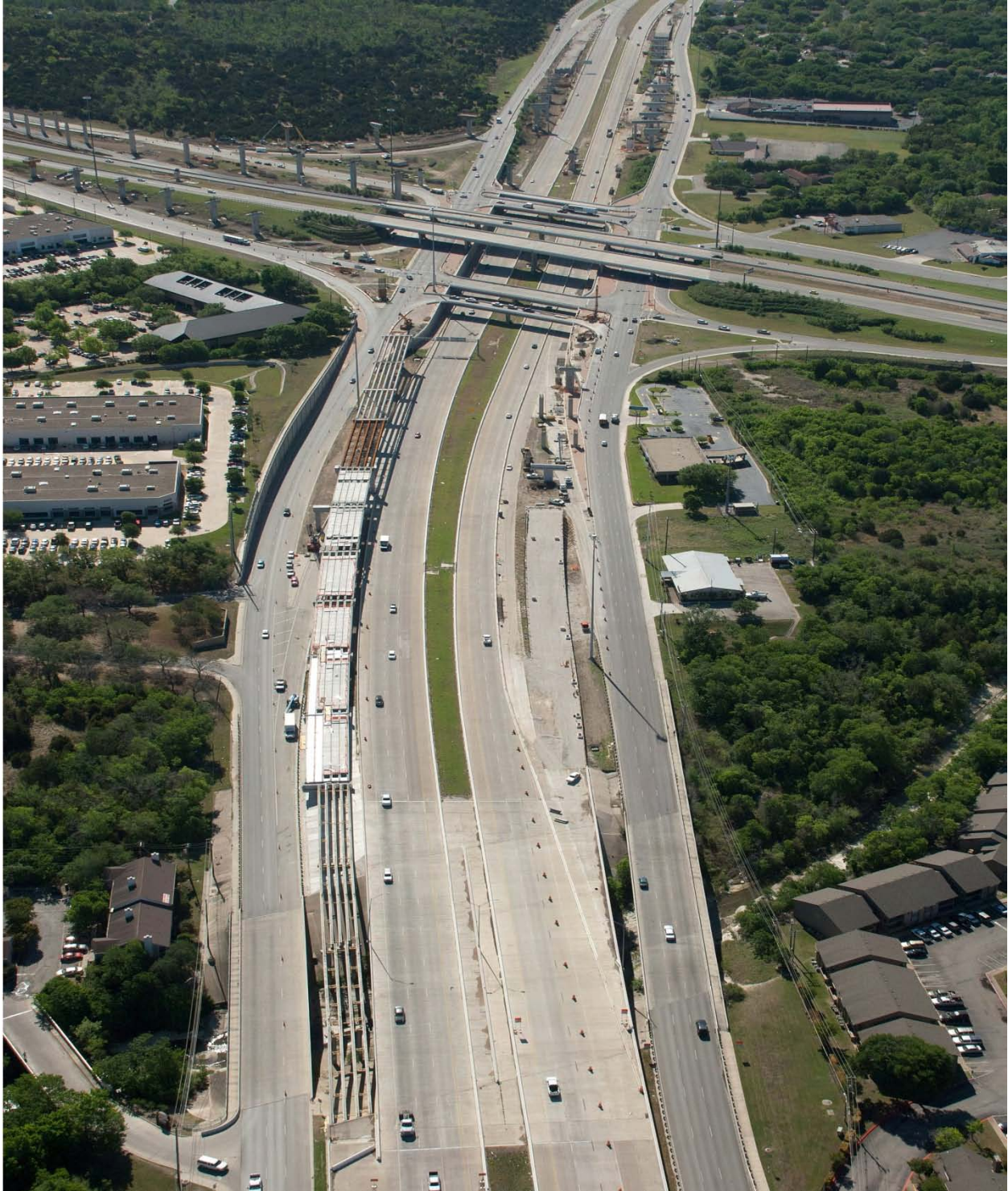
Interchange construction looking south (Taken 4/11/2011)
