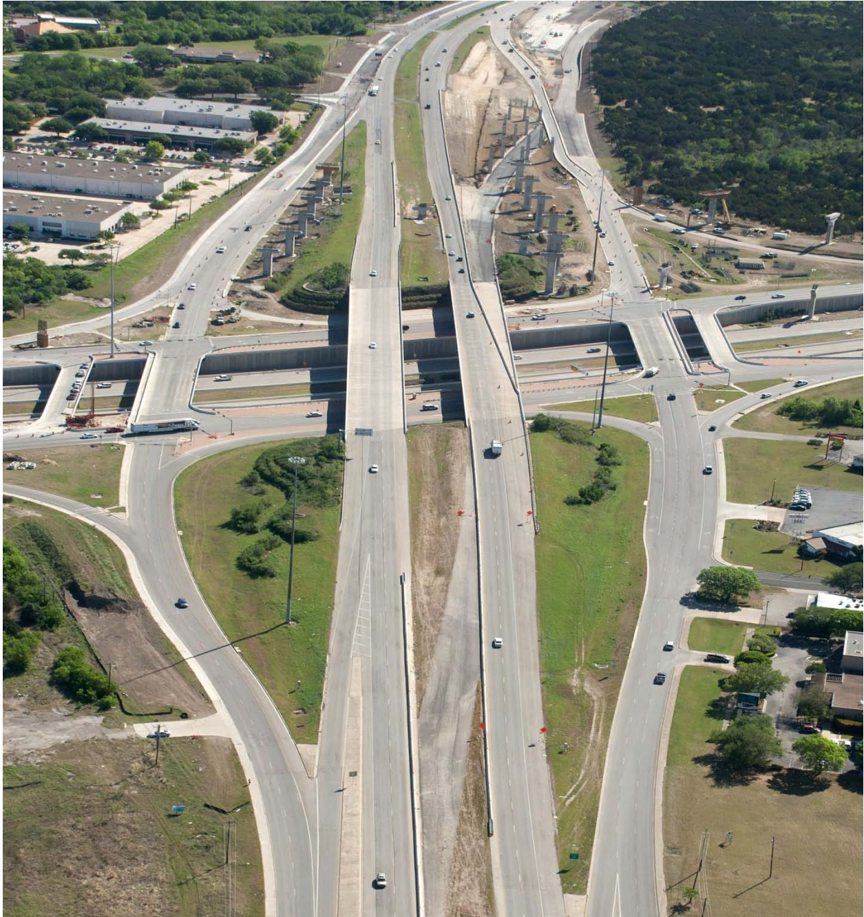
Interchange construction looking east (Taken 4/11/2011)
