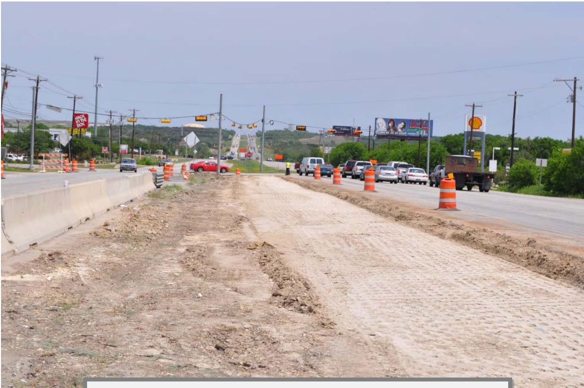
Earthwork near Tuscany Way intersection (Taken 4/14/2011)
