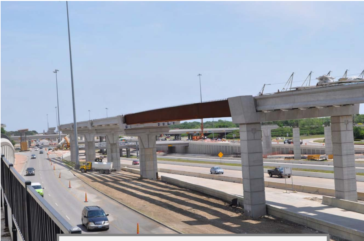
Beams at west to north direct connector (Taken 4/14/2011)
