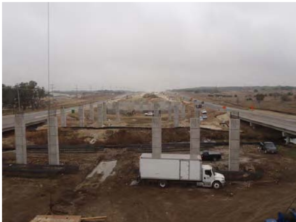
Bridge columns at RM 2243, looking south
