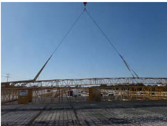
Preparations for placing concrete on a bridge deck at New Hope Drive
