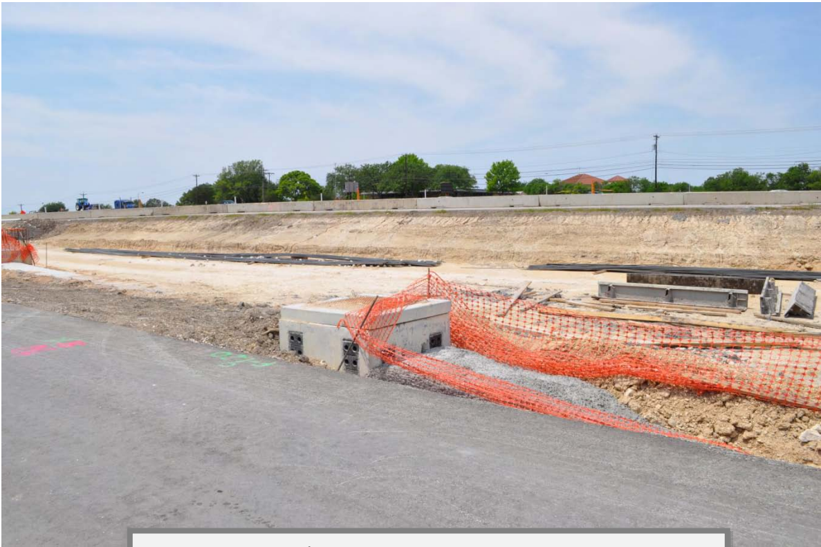
Roadway appurtenance construction (Taken 1/14/2011)
