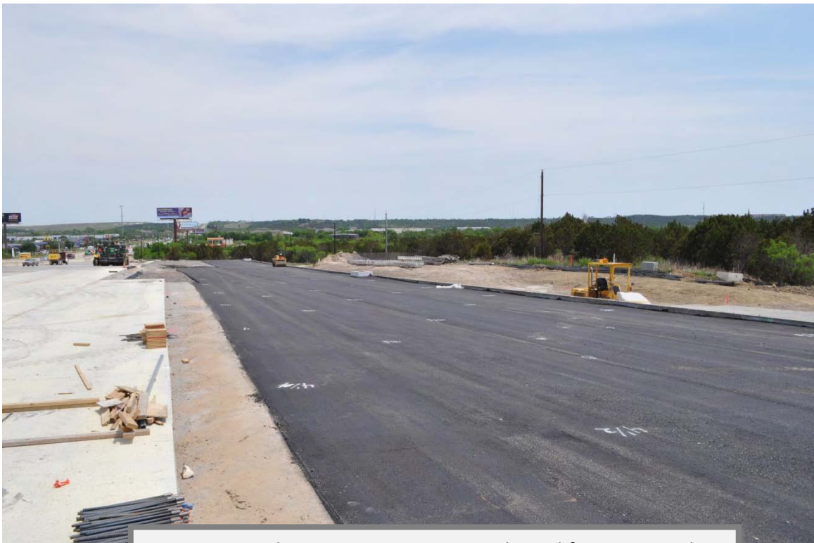
Pavement base construction at eastbound frontage road (Taken 4/14/2011)
