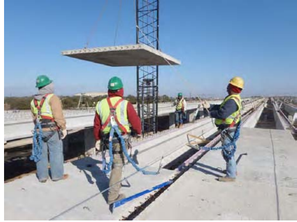
Setting deck panels at New Hope Drive
