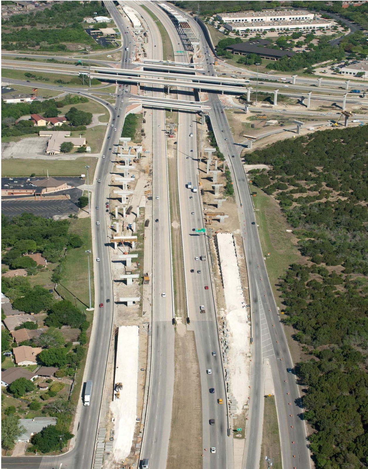
Interchange construction looking north (Taken 4/11/2011)
