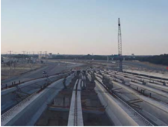
Preparations for setting deck panels at New Hope Drive
