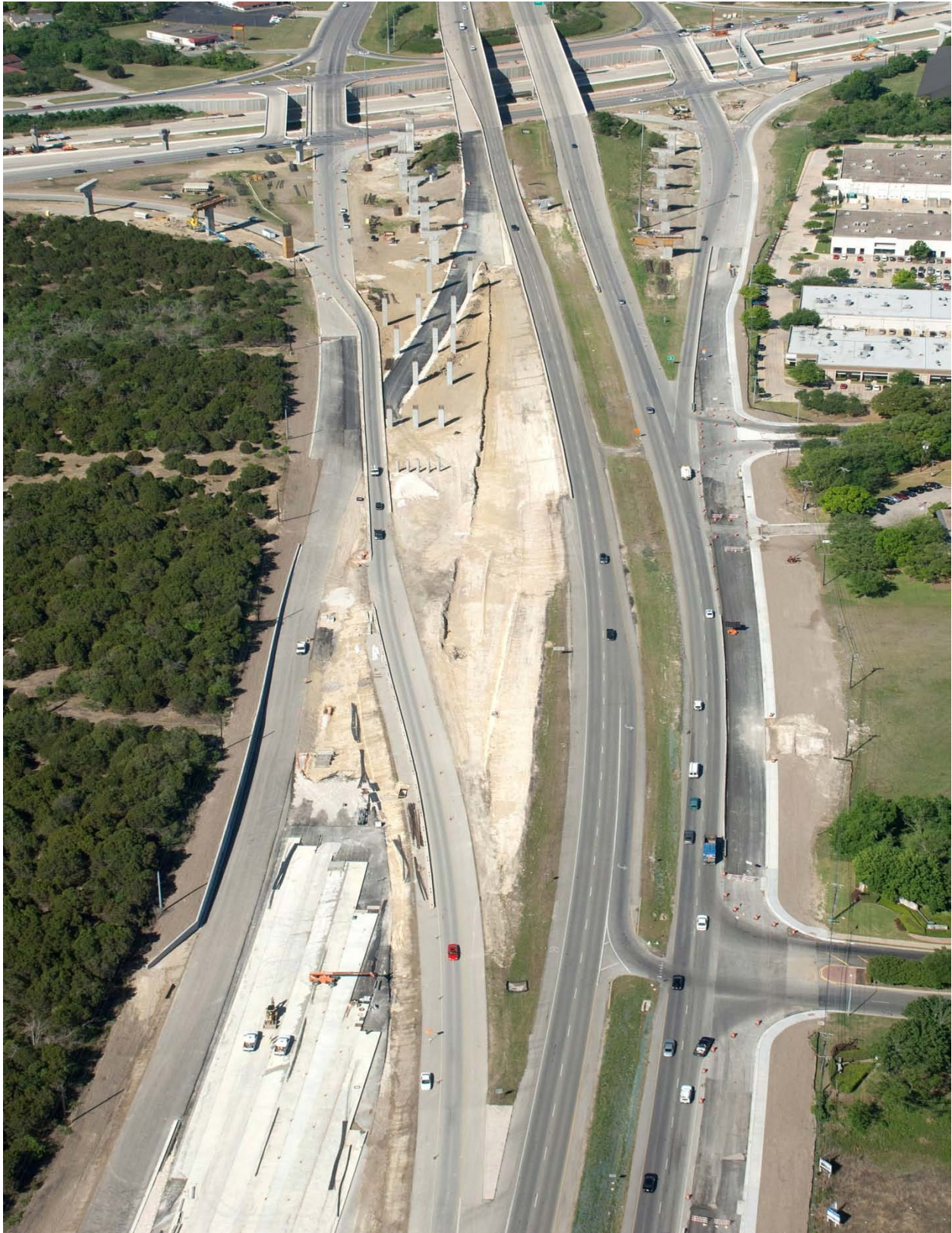
Interchange construction looking west (Taken 4/11/2011)
