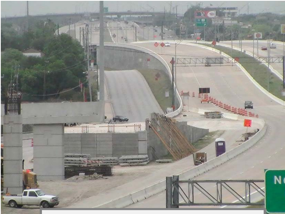
Direct connector abutment construction (Taken 4/14/2011)
